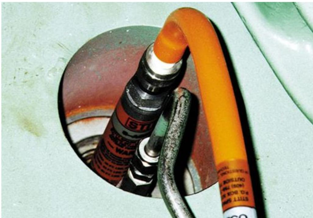
What is the problem? Plastic does not retain its original dielectric [high-voltage insulating] proper-
